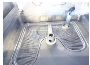
Replace the overflow pipe
